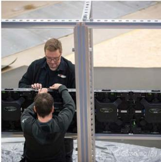
▲ Fixing the LEDskin® frames to the beMatrix aluminium frames is easy with the handy standard M8 connectors. Ready in a jiffy and always firmly and securely anchored.
